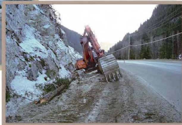
Following a post-blast inspection, blasted rock is removed.
