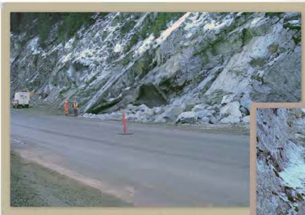
Following a post-blast inspection, blasted rock is removed.
